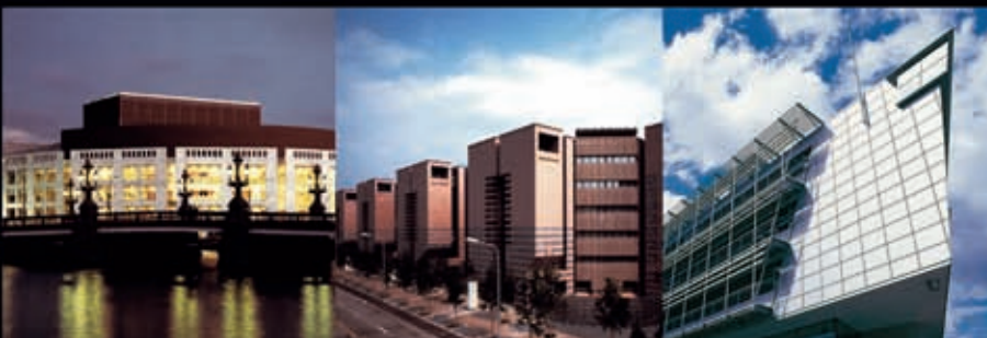
City Hall, Amsterdam NL Banca del Gottardo, Lugano CH Titanic-Building, Bern CH
